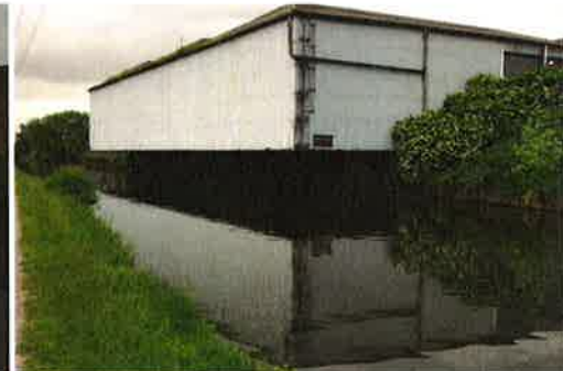
Disused loading bay
