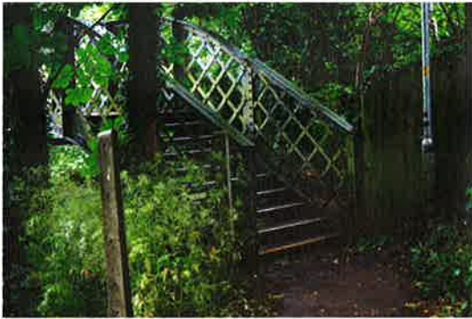
Footbridge at Broxbourne
