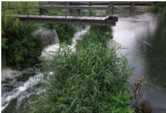
Dobbs Weir is an unusually complex piece of engineering: the vertical overfall is not the usual straight span but in plan is closer to what is known as a ducks bill weir, where the water falls into a series of slots, making the surface area that it drops over greater. The purpose of this could be to facilitate higher volumes of water when the river is in spate. This is hugely overgrown with semi-mature
